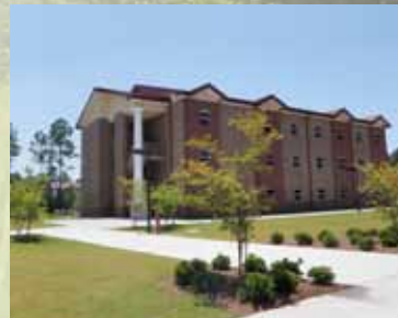
EAB BARRACKS | LEED SILVER
