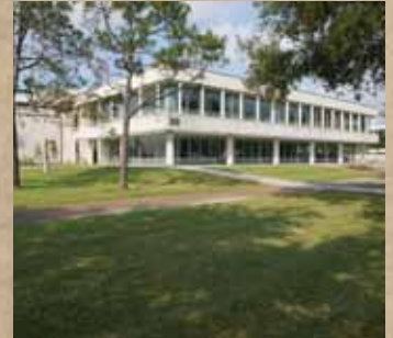
BUILDING 29 FOR CEV AND CAIL | LEED SILVER
