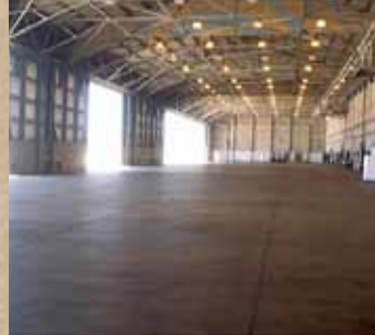
REPAIRS TO HANGAR A-981 | LEED CERTIFIED
