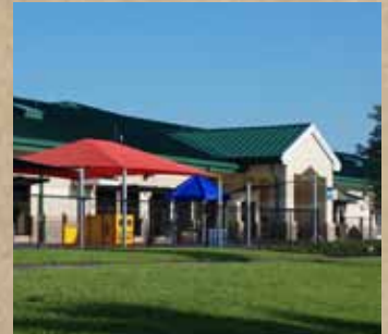
NAS JAX CHILD DEVELOPMENT CENTER | PENDING LEED GOLD
