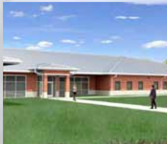
SPAWAR ELECTRONIC INTEGRATION & SUPPORT FACILITY
